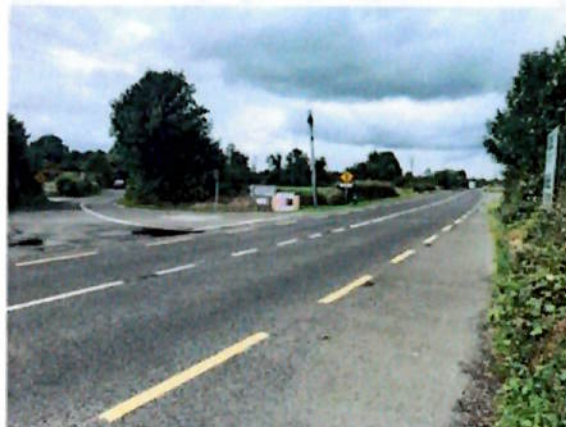
Photo 05: View to the north illustrates the continuous white line and road alignment.
