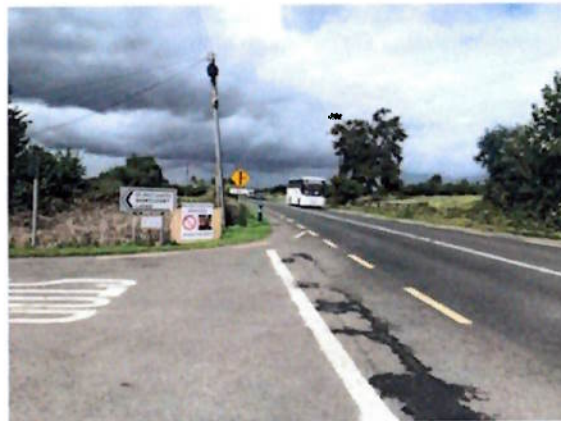
Photo 02: View to the north with hedging and signage and other road furniture impeding the sight line.
