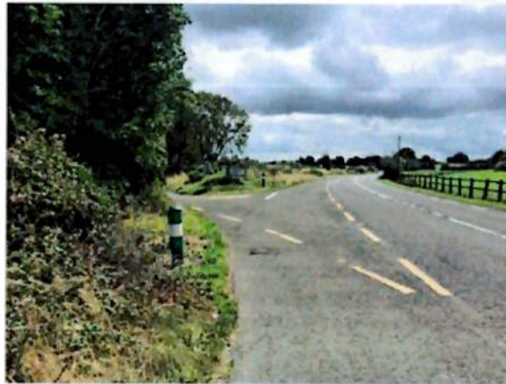
Photo 04: View to the south illustrates the curvature of the road and fence limiting the sight line from the road junction.
